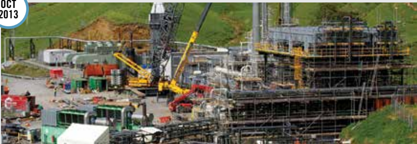
Site construction nearing completion
