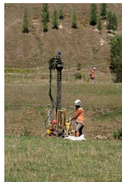
Helicopter Seismic Drilling Rig
