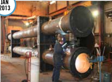
Fabrication underway at Propak, Calgary
