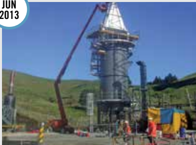
Hot oil heater installation
