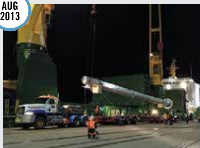
Unloading Propak equipment at Port Taranaki
