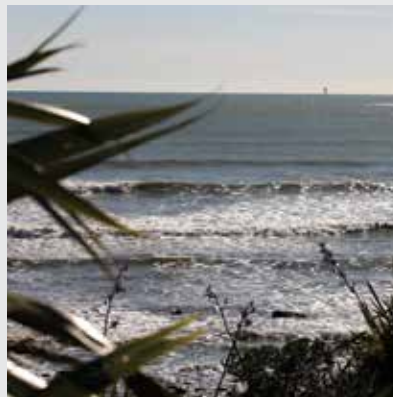
Remote operation of Production Station. Pohokura in the distance.
