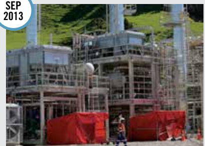
Building the plant - ractionation area
