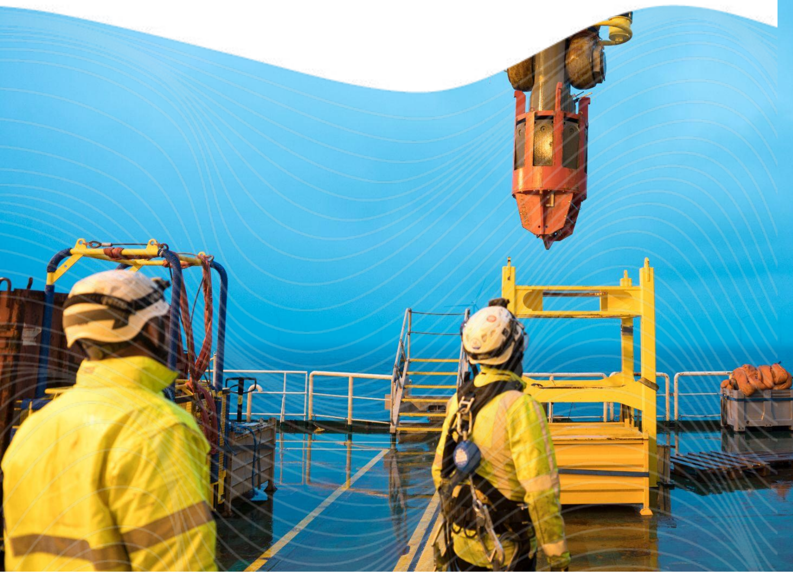
Image: Installation works for Northwester 2, Belgian North Sea, Courtesy of Parkwind.
